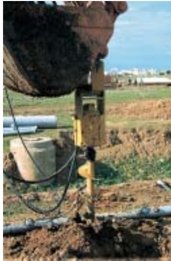
Cantiere Gloulou Tunisi Gloulou job-site - Tunisia chantier Gloulou - Tunisie
